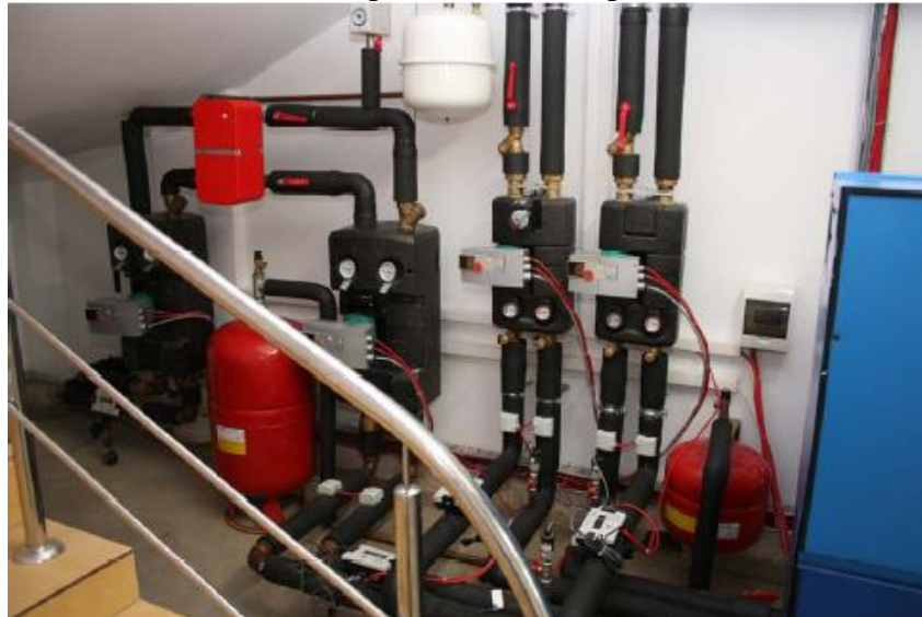
Picture 2 Chiller pumps station
